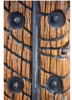
Reinforcement High Acceptance Ian Hughes
